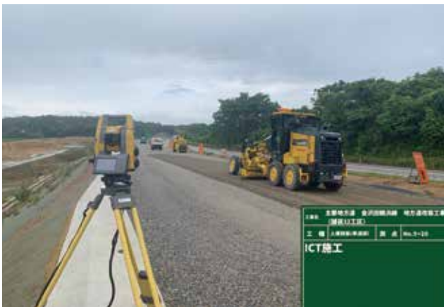
ICT 建機での敷均し
